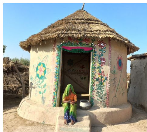
Flood resistant, prefab bamboo LOG built on lim/ brick and lime/concrete foundations.
