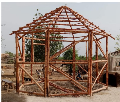
Flood resistant, prefab bamboo LOG built on lim/ brick and lime/concrete foundations.
