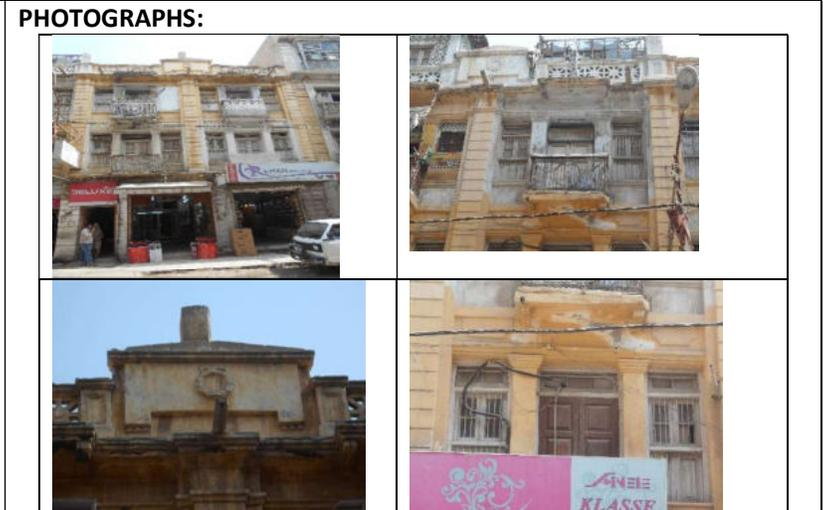
**11. COMMENTS:** *Building is partially maintained. The Extra additions and alterations including untidy electric wires and hoardings need to be removed.*
